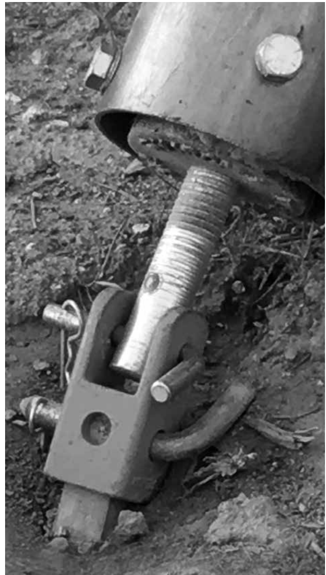
INCORRECT Brace-to-HGA Connection
